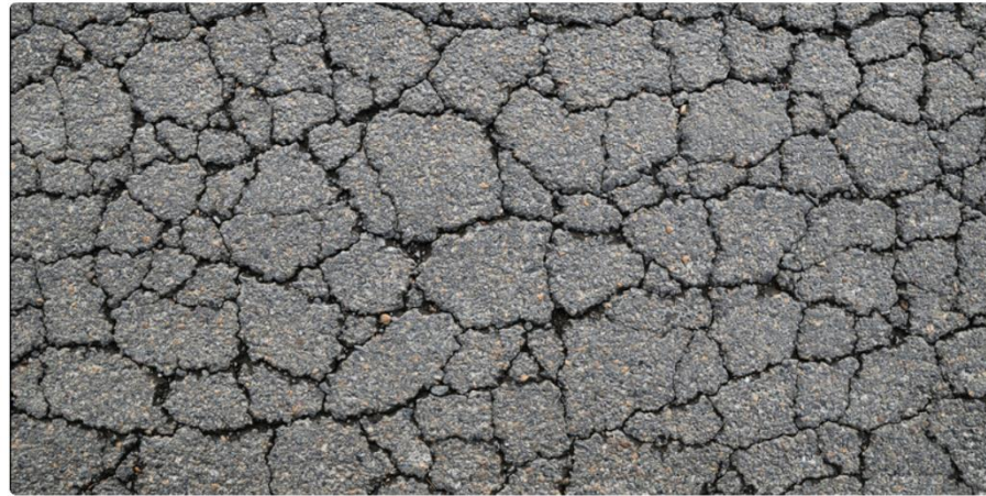
Fatigue cracking
