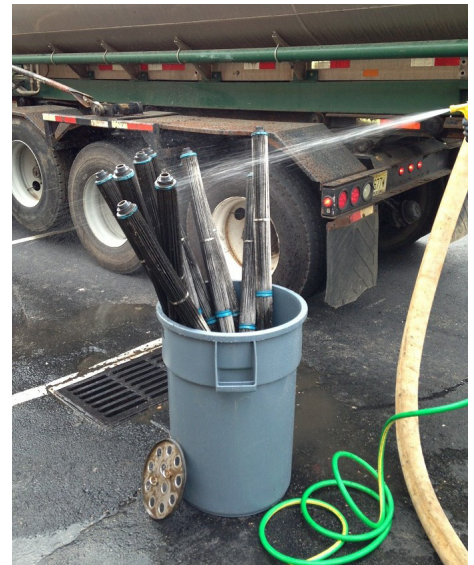
Rinsing of dirty filter cartridge tentacles with a low-pressure garden hose sprayer, and using a plastic garbage container to capture rinse water.
