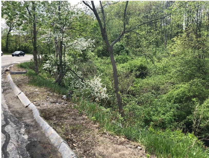
FIGURE 5 Looking south into brush and College Brook.
