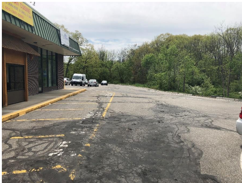
FIGURE 4 Looking south in front of existing building.
