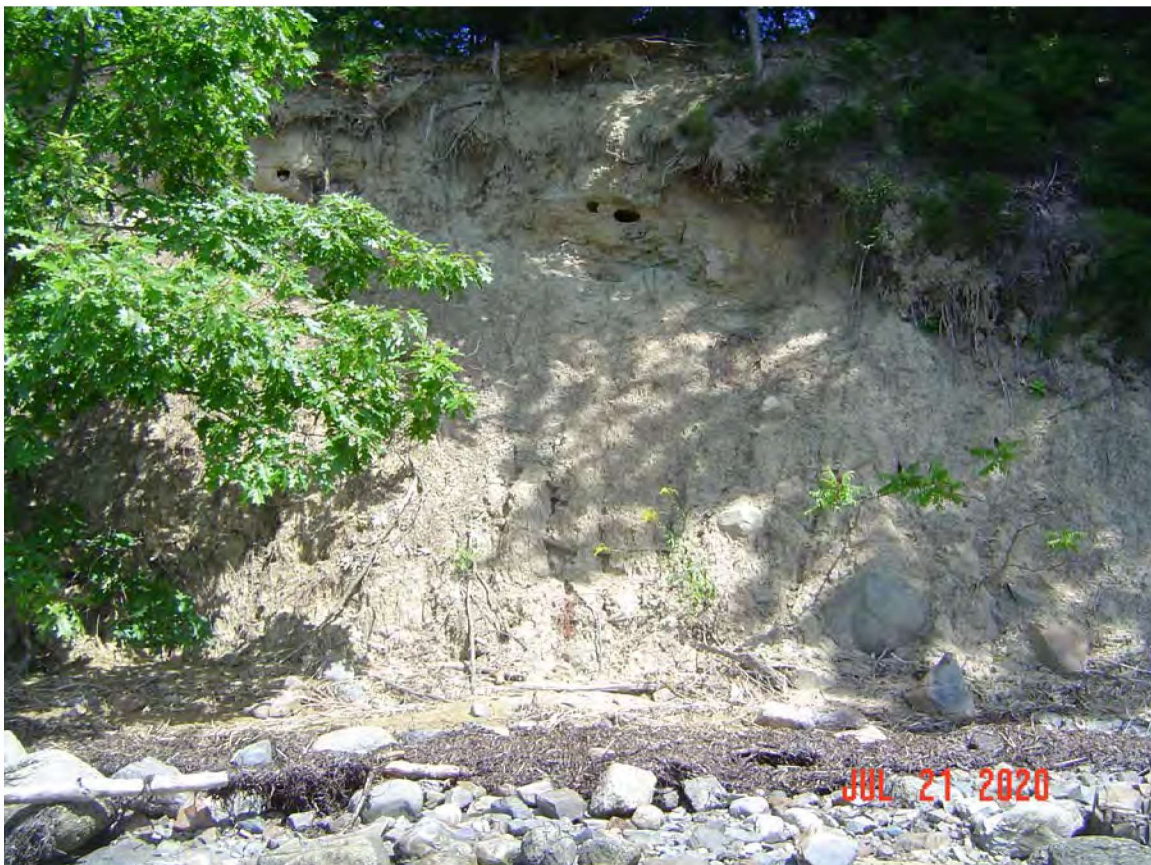
Image 12 – Looking north at low tide at the south side of Fox Point in Newington. Note the severe bank erosion. The distance from the wrack line at the bottom of the image to the top of the bank is approximately 20+ feet. Note the bird nesting cavities near the top of the bank. (©Jacobs2020)
