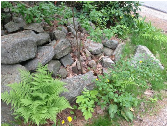
Existing opening for driveway; cast aside stone wall we will restore.
