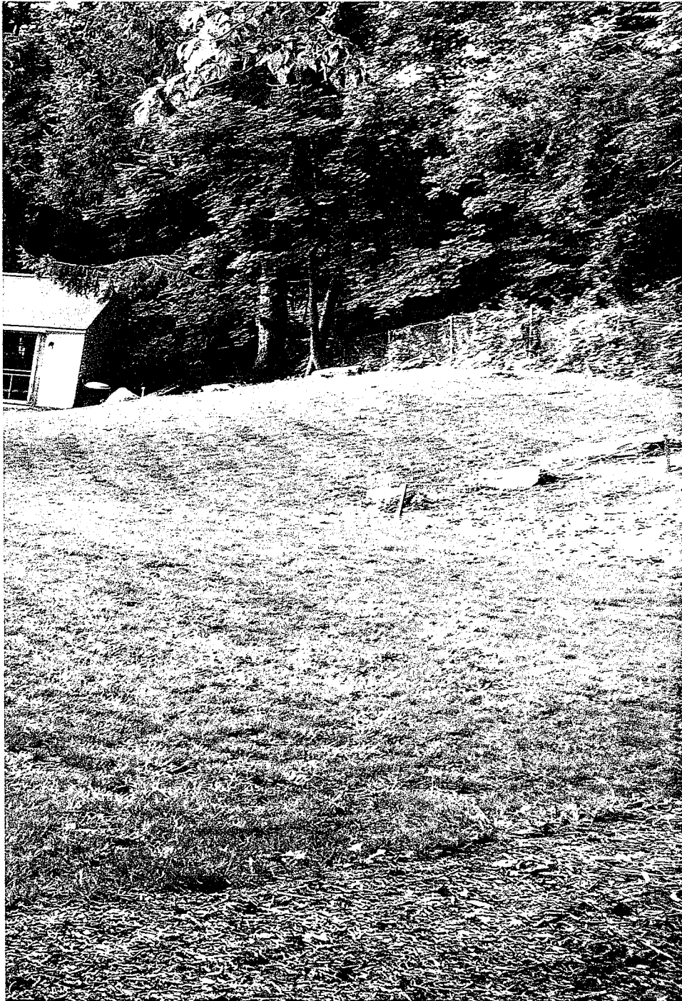
View from back wall looking toward back of home. Chain link fence showing vegetation and damage from falling trees evident.
