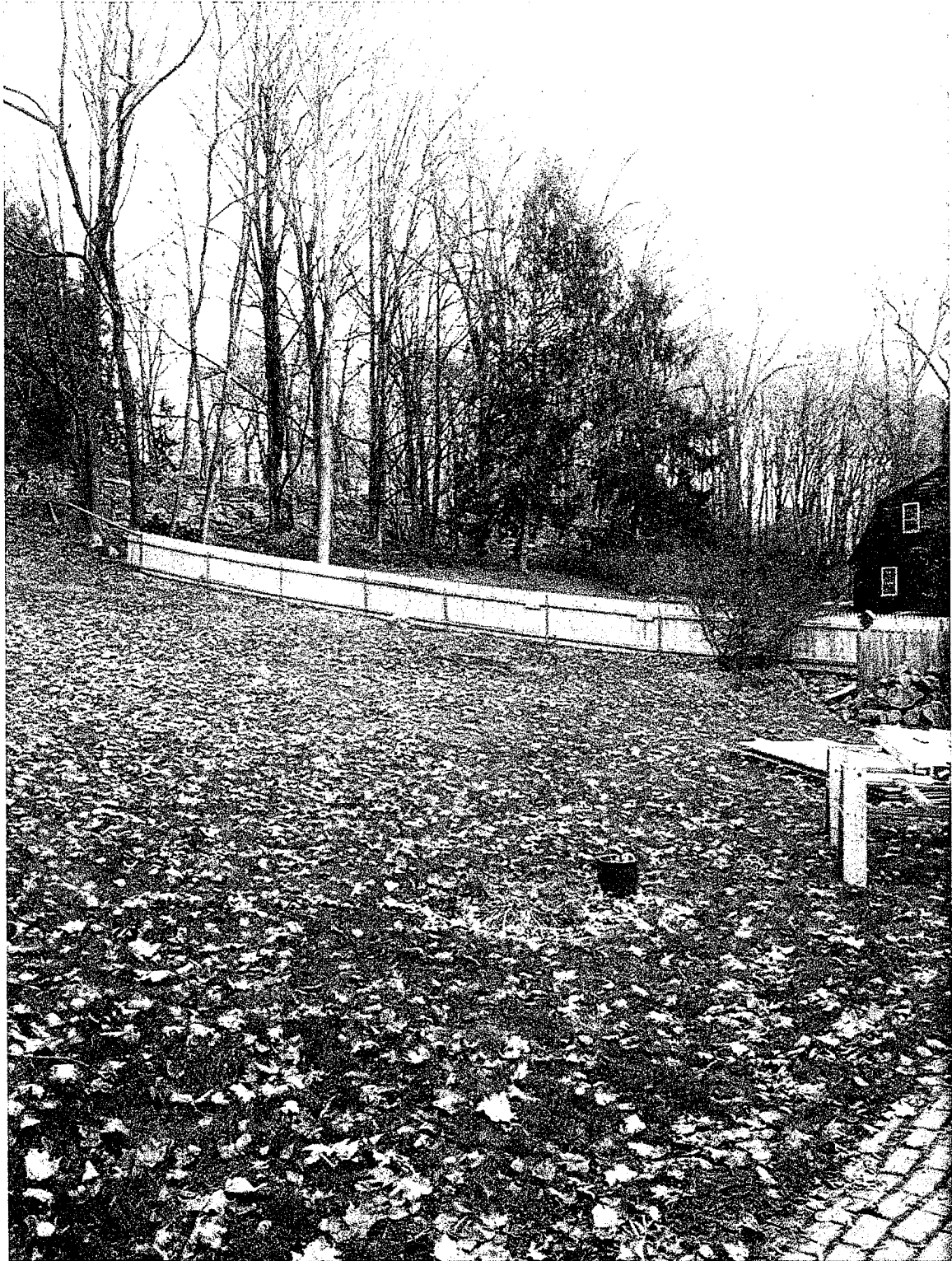
Similar view from home toward Moriarty with fence nearly completed.
