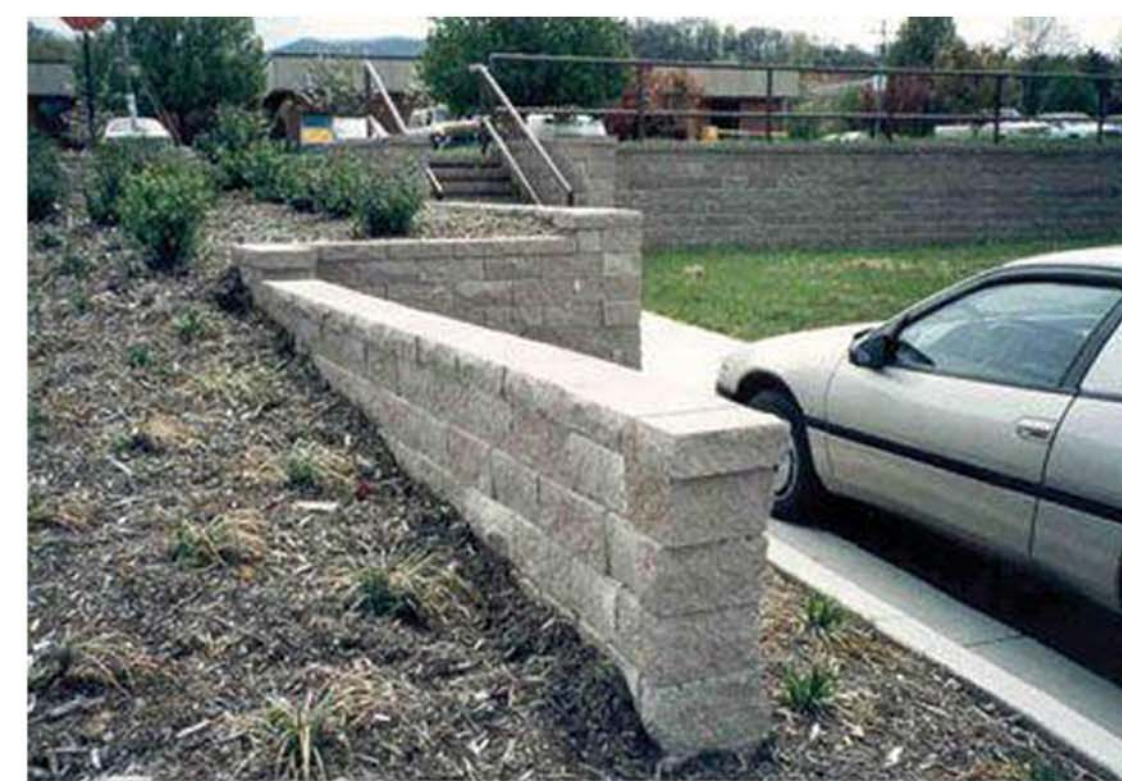
EXAMPLES OF VERSA-LOK RETAINING WALL
