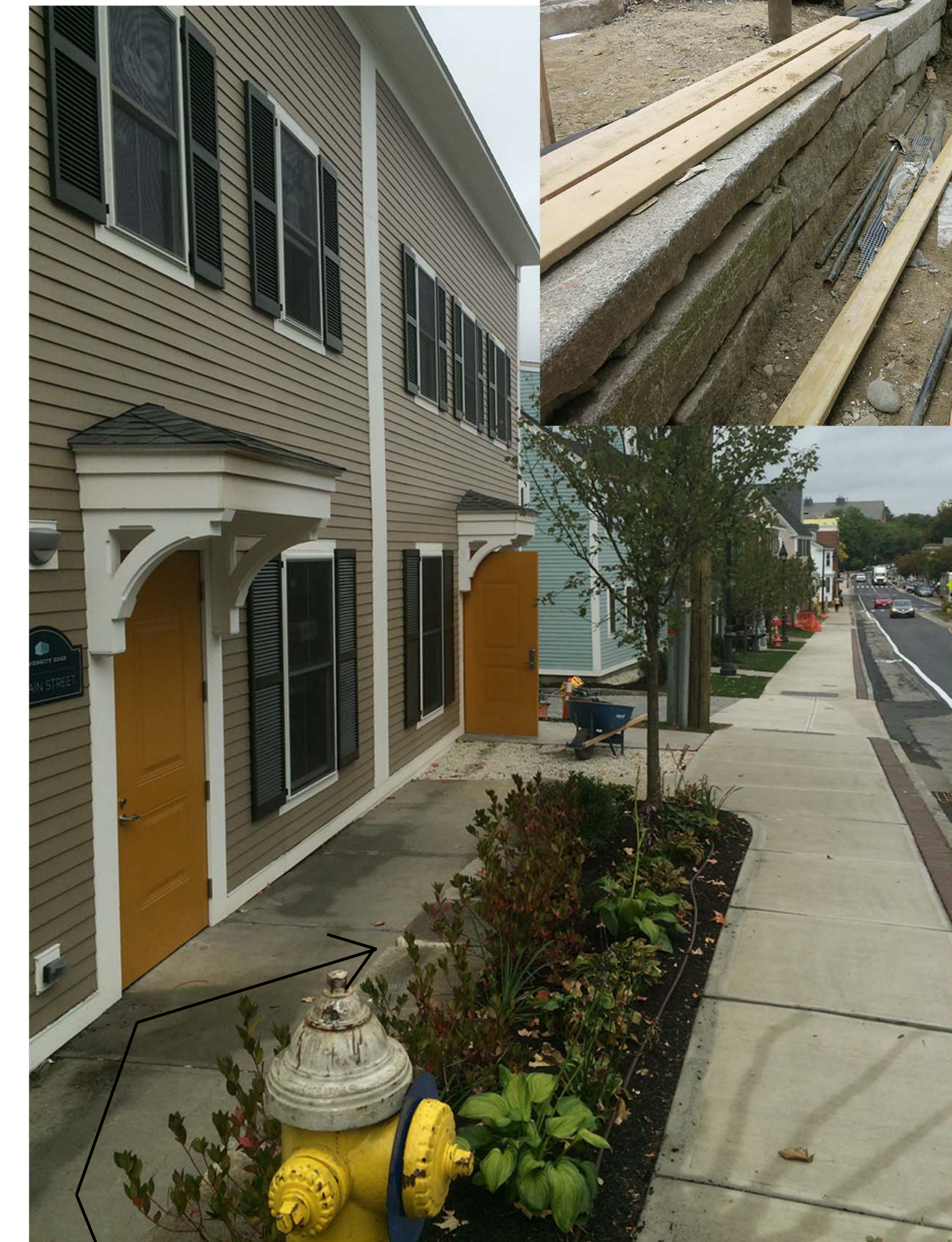
VIEW FROM MAIN STREET SIDEWALK
