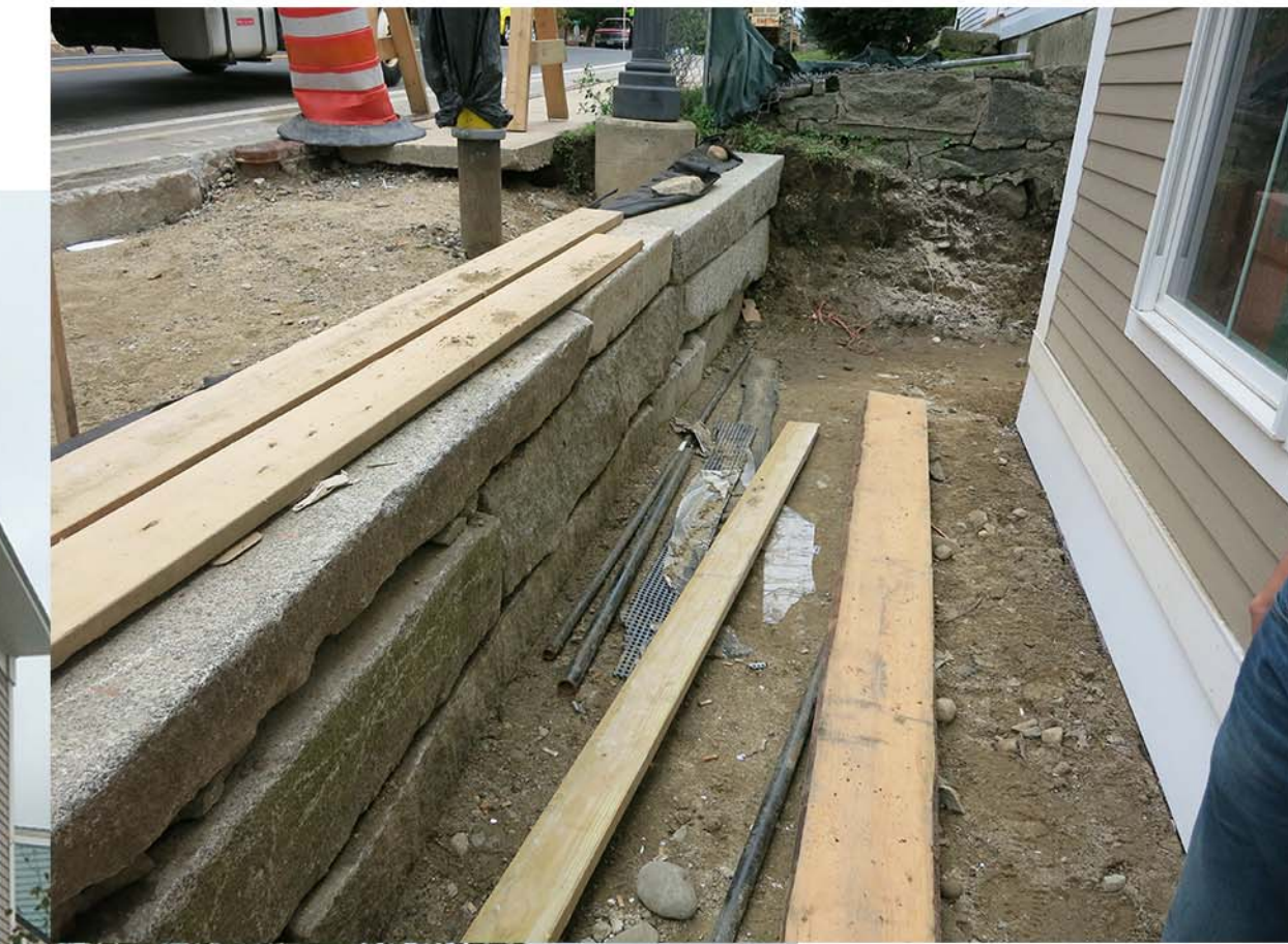
VIEW FROM INTERIOR WALKWAY
