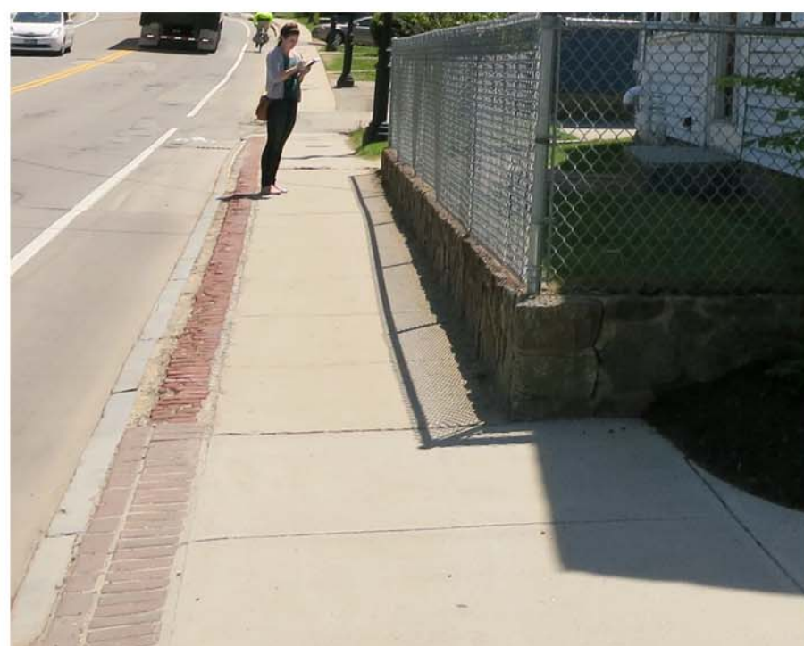
OLD STONE WALL
