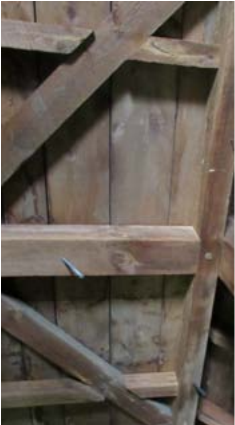
Existing Barn Sheathing
