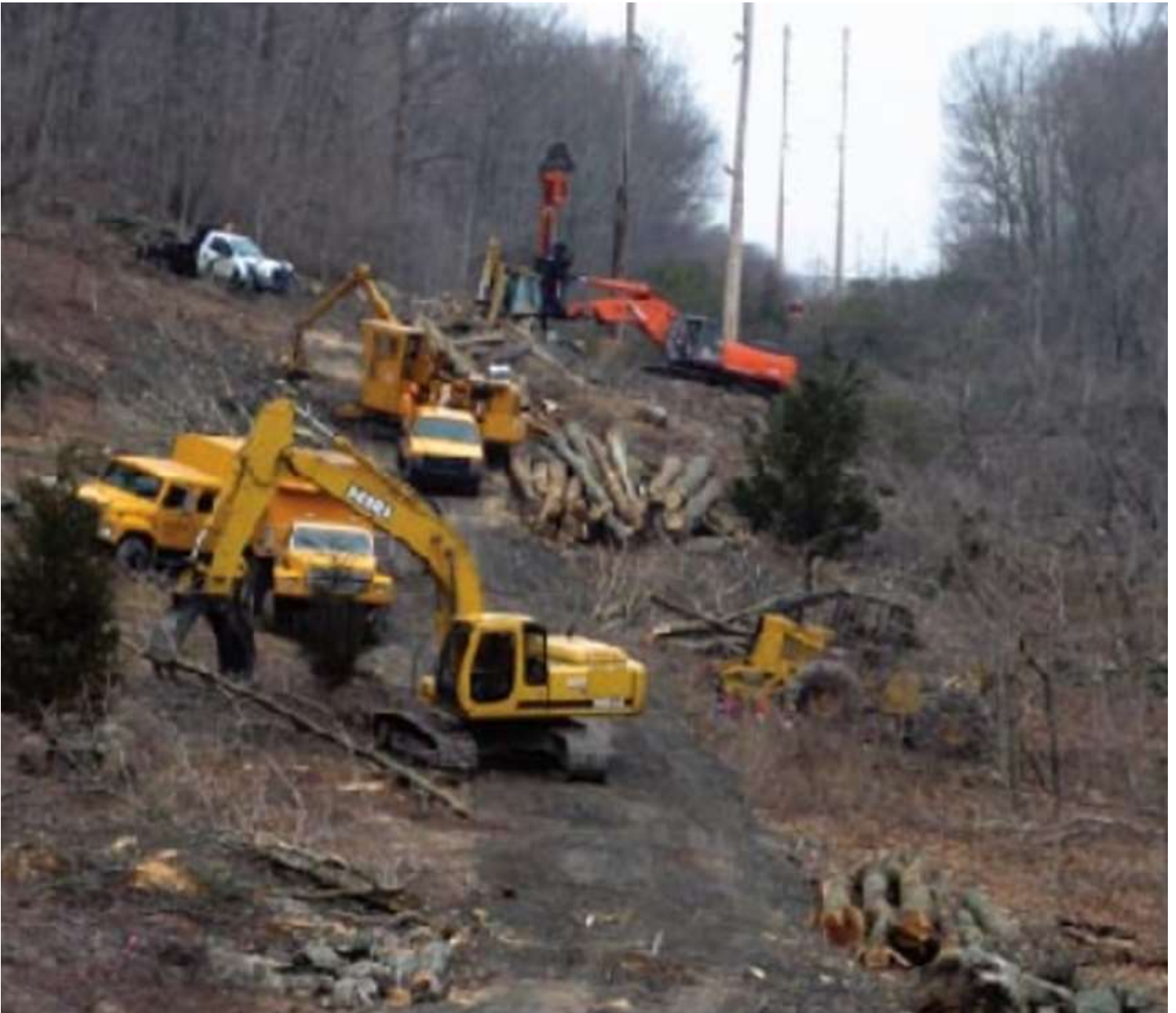
Job site with typical equipment spread across easement, from Eversource website
