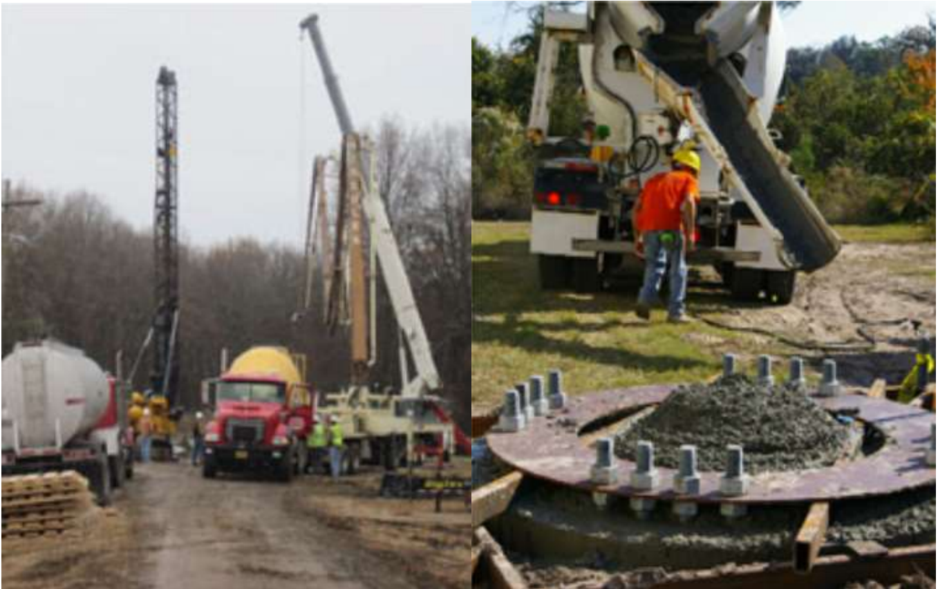
Concrete trucks at pylon installation site
