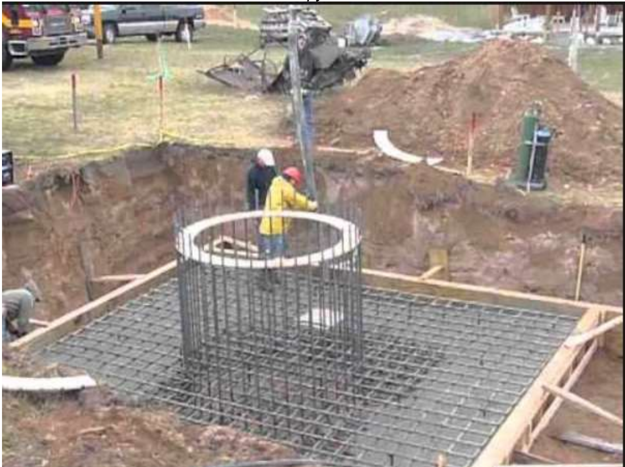
Reinforced pole base
