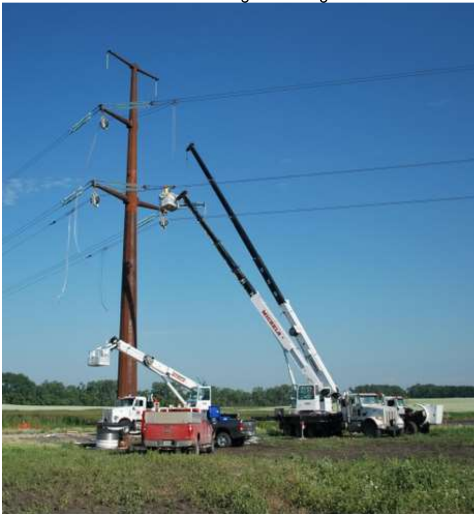
Multiple cranes at job site
