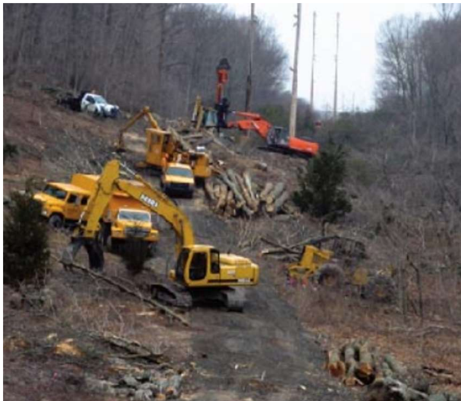
Image 55: Erecting pylons in New Hampshire, from the Eversource website
