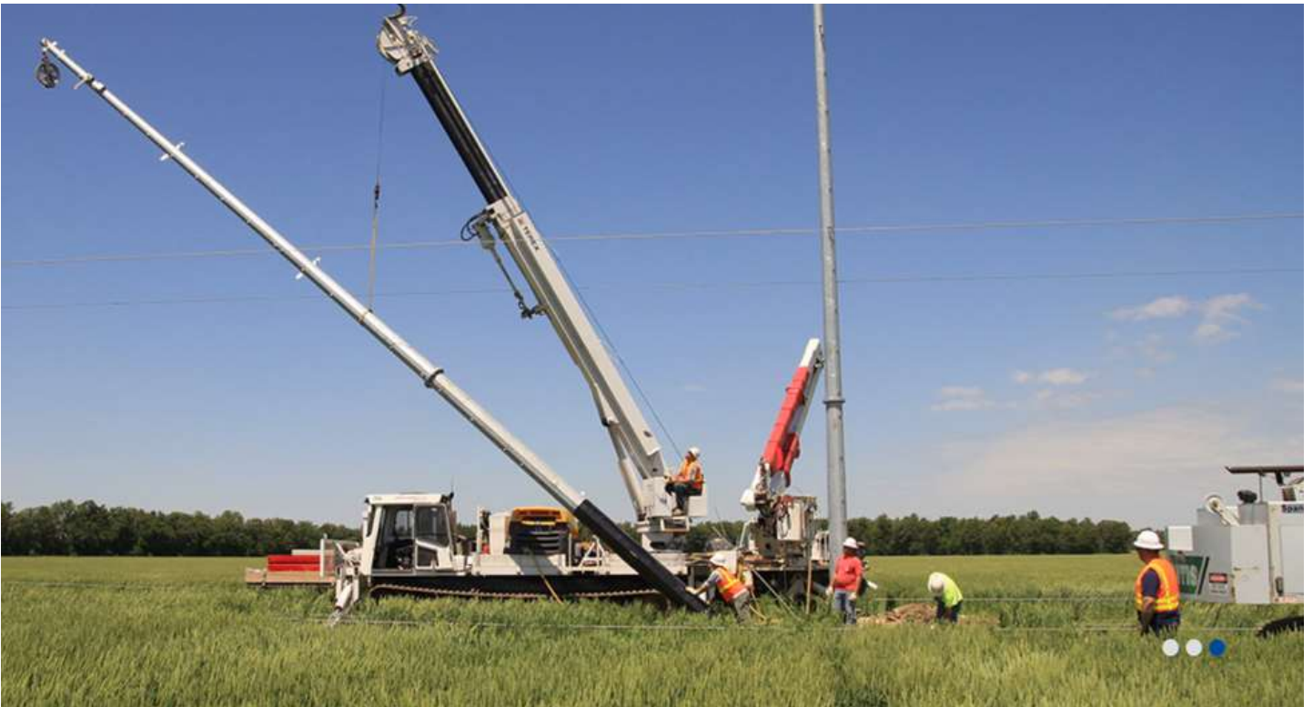
Crane on tracks maneuvering assembled pylon
