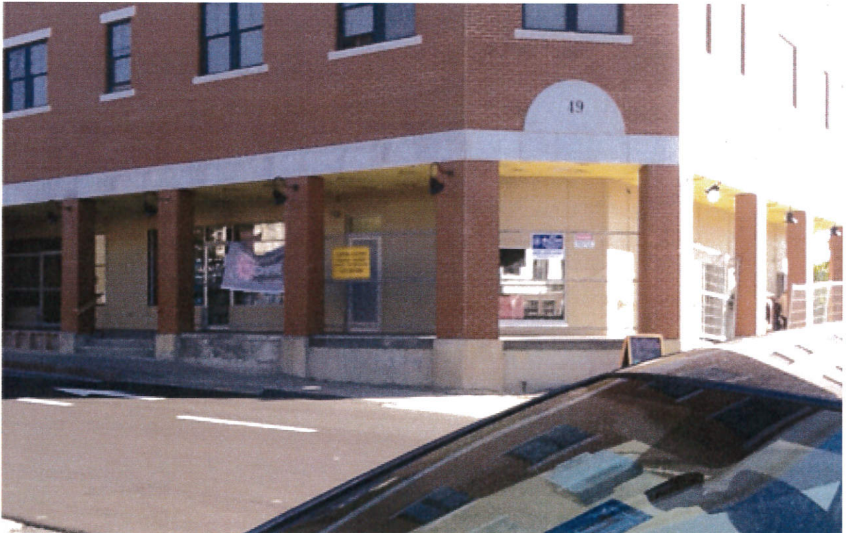
October 6, 2015 — Finished lunette installed
