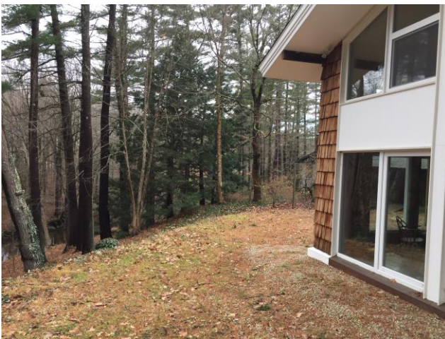
Rear of house. Stone terrace to be installed
