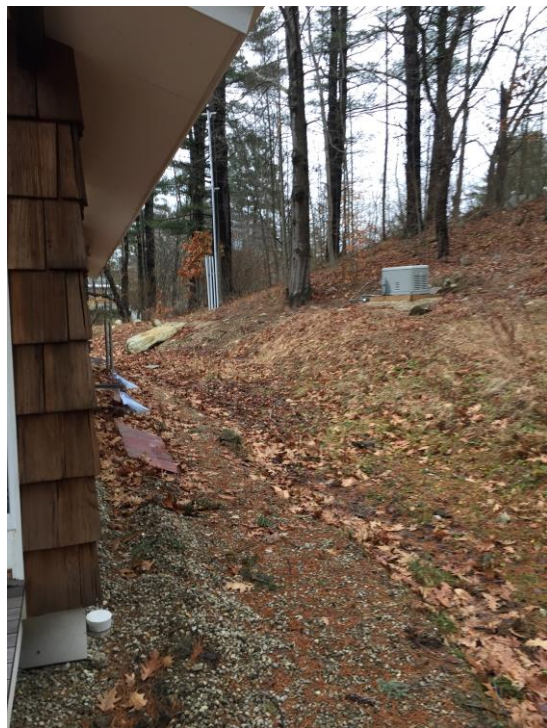
Easterly side. Ditch to be laid with rip rap
