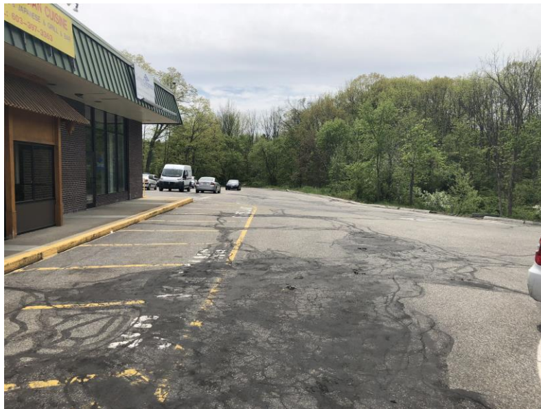
FIGURE 4 Looking south in front of existing building.
