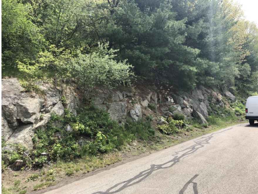
FIGURE 9 Looking southeast at rock ledge behind second existing building.
