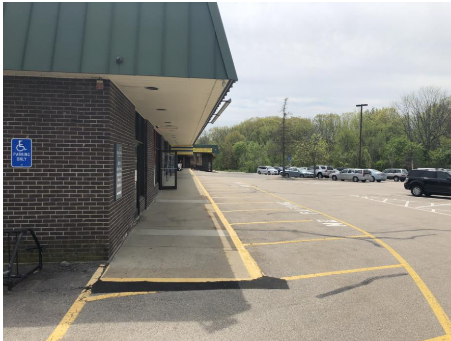
FIGURE 11 Looking south down the second existing building.
