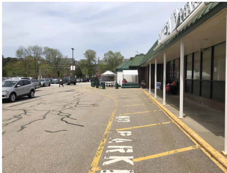
FIGURE 14 Looking northwest towards Mill Road.
