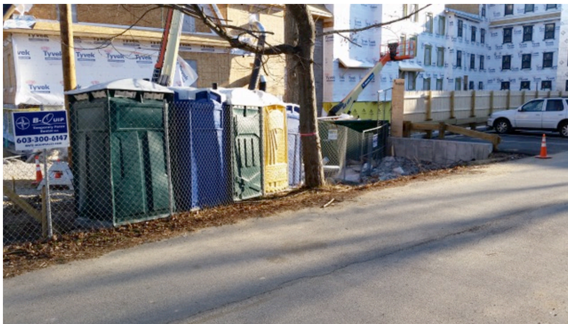
2014: tree unprotected during construction
