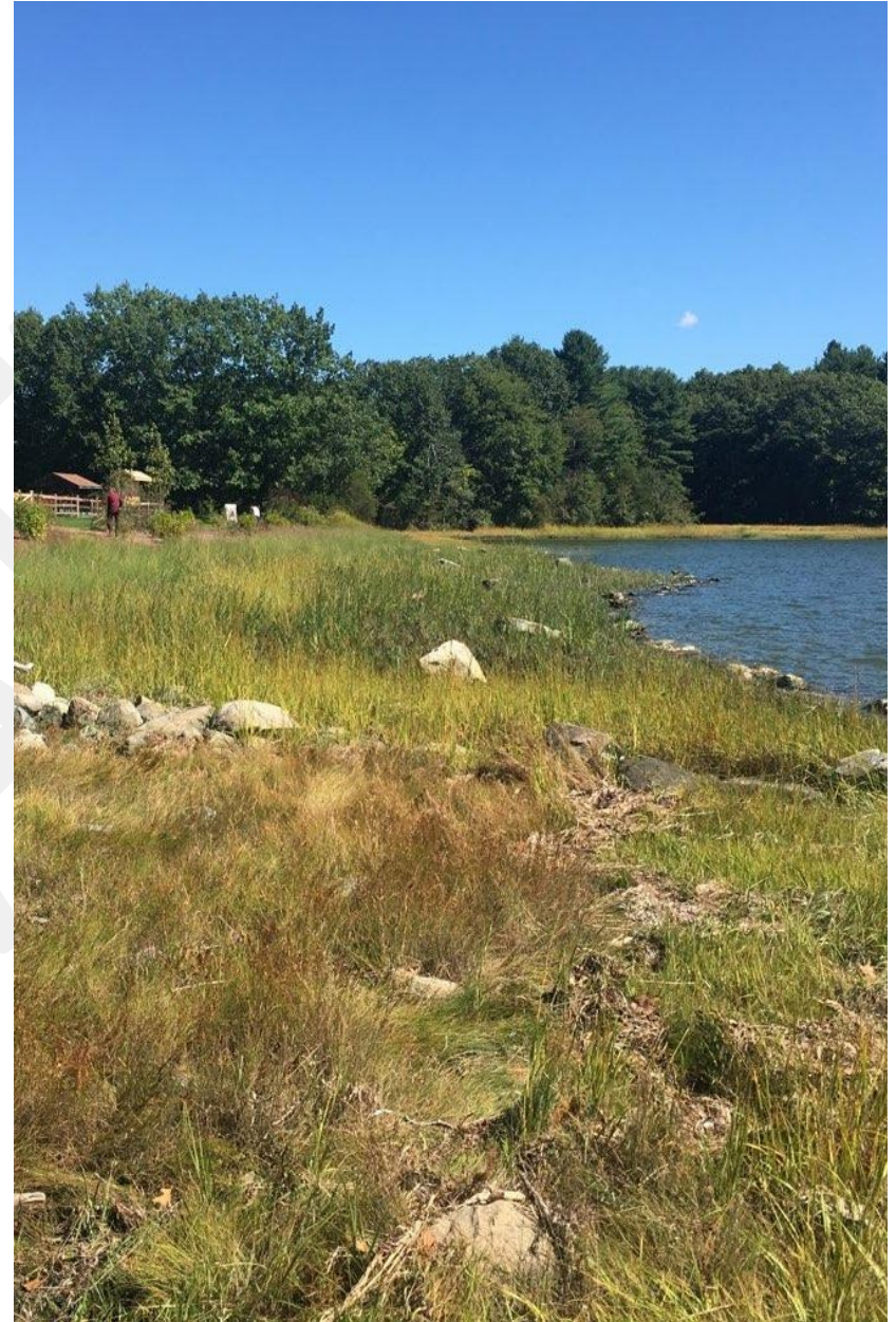
Living Shoreline Installation at Wagon Hill on Great Bay (Photo Credit: NHDES)
