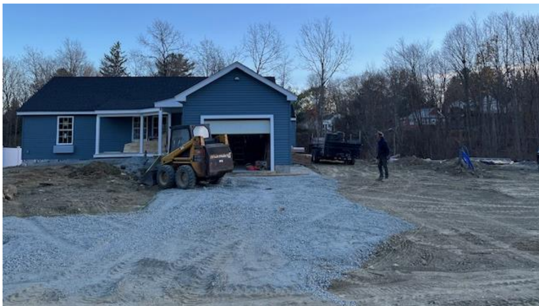
Lot 92. Under construction. Right side to be built:
