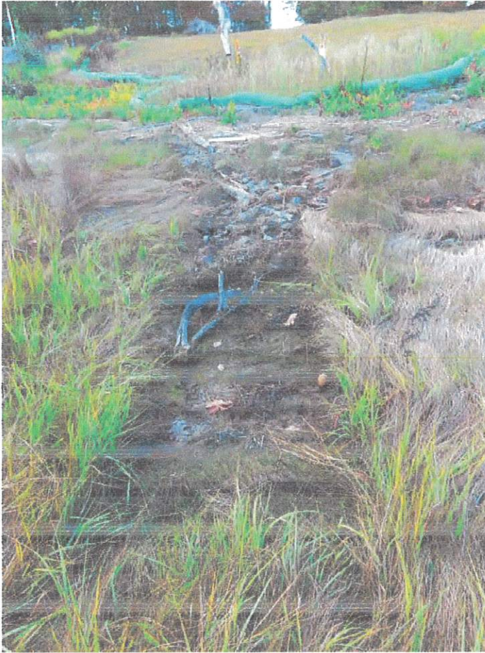
57 TON EXCAVATOR DRIVEN ON THE SALT MARSH WITHOUT TIMBERMATS. CATEPILLAR TRACKS MARK DEAD AREAS OF SALT MARSH. SILT SOCKS/DEBRIS REMAINING ON LAND
