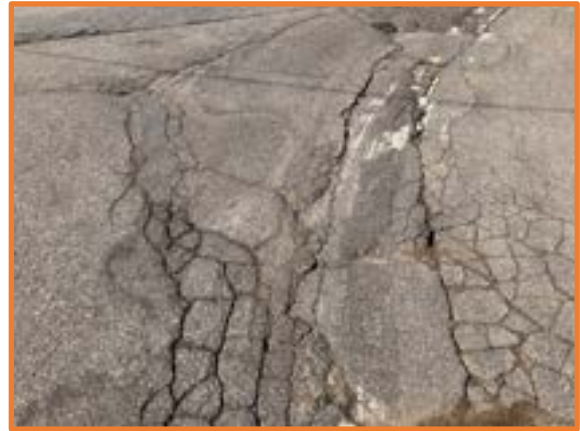
Dennison Road with severe alligator cracking indicating roadway base failure
