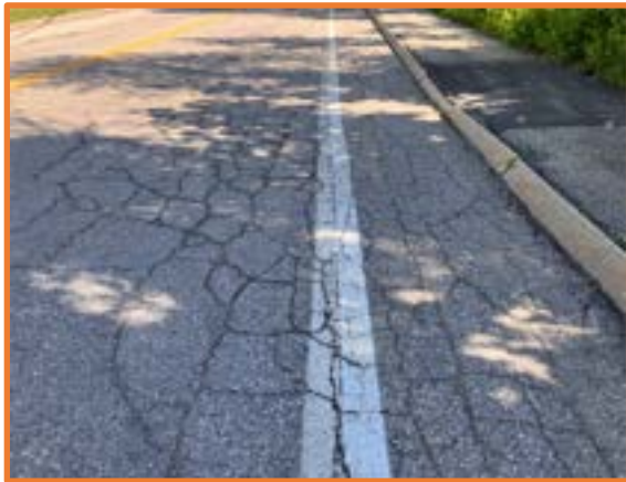
Dennison Road with severe alligator cracking indicating roadway base failure
