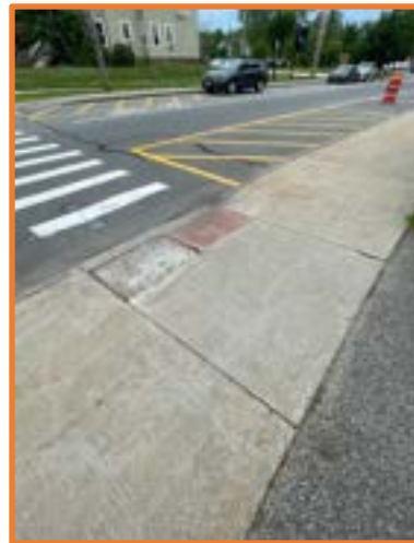
Main Street and Pettee Brook Sidewalk Panels requiring repair
