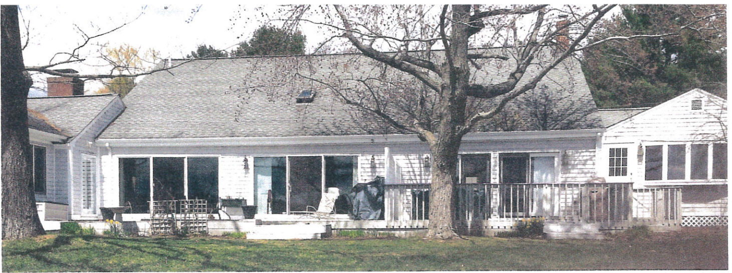
Current Deck Picture Taken 2/26/15
