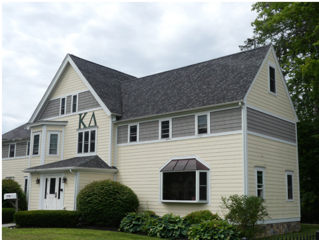
Photograph 2: Kappa Delta Northeast Elevation
