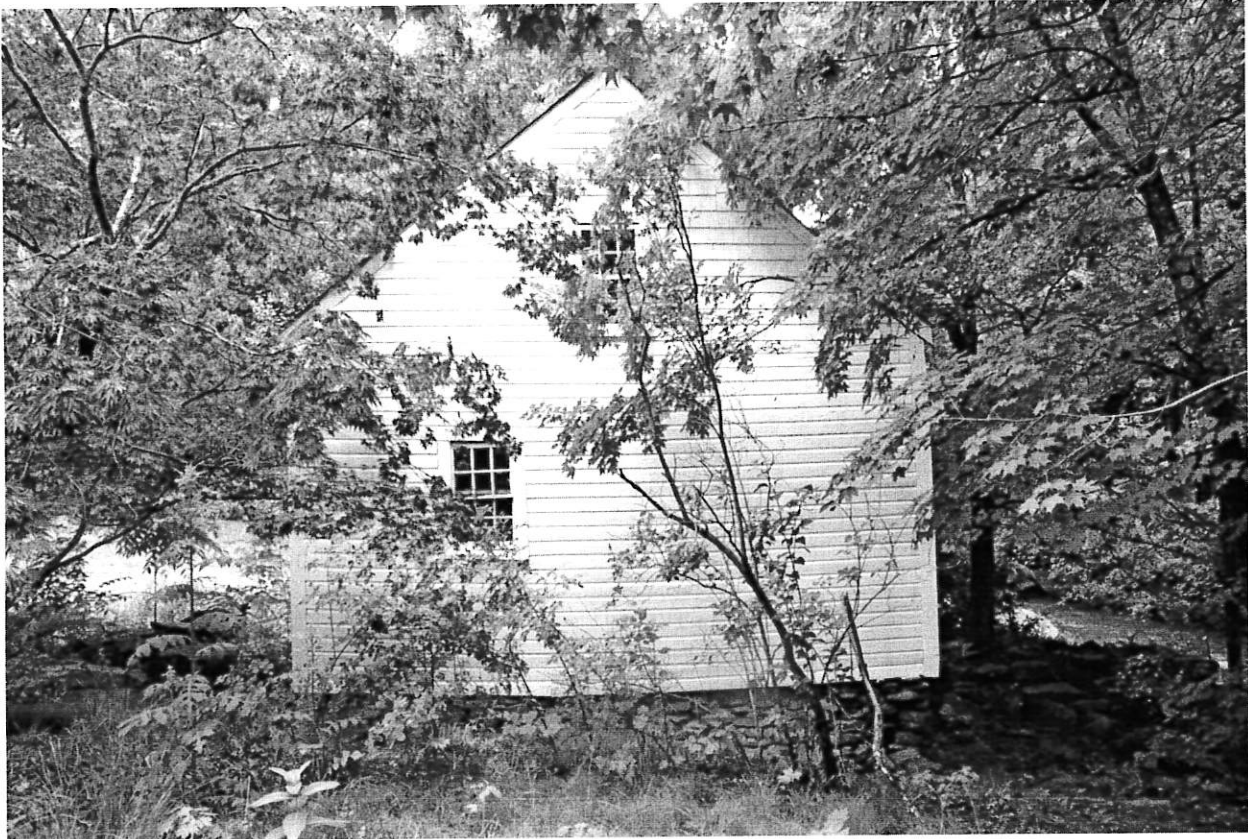
Elevation – Southeast (facing Mill Road)
